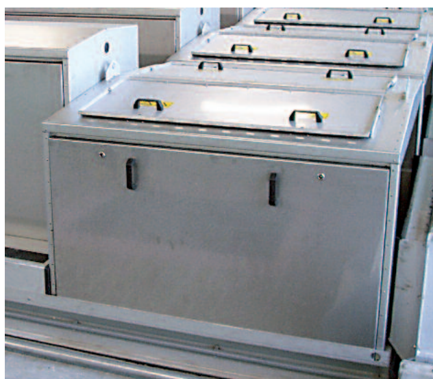
Parallel installation of several HUBER Curved Bar Screen CurveMax® units with odour-tight covers
