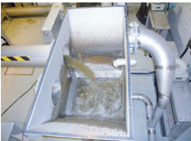
The flushing water serves also as wash water.
