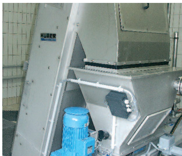
Rear view of a HUBER RakeMax® Screen with subsequent Wash Press WAP/SL
