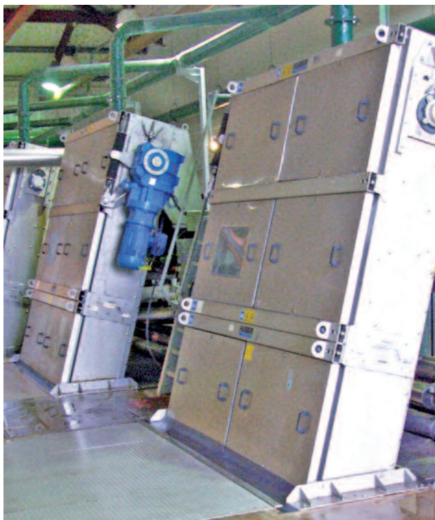
Universally applicable HUBER RakeMax® screen for big channel widths ...
