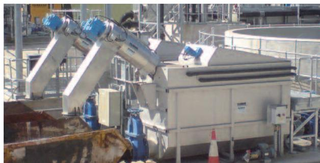
*ROTAMAT® Membrane Screen RoMem units in tanks*
