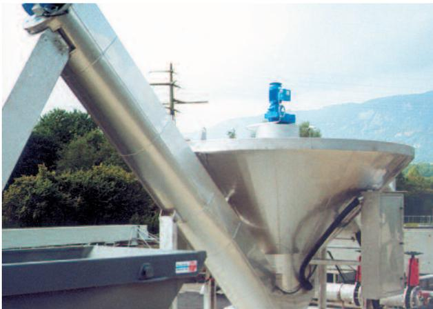
*Innovative technology: HUBER Coanda Grit Washer RoSF4 size III with frost protection for outdoor installation*
