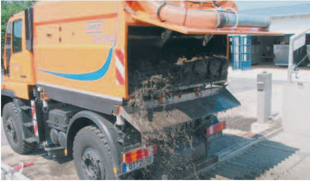
Acceptance tank with bar grate and integrated horizontal dosing screw
