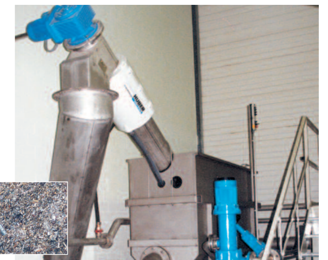
ROTAMAT® fine screen for 1 mm screening and dewatering of organic material (approx. 30% DR)
