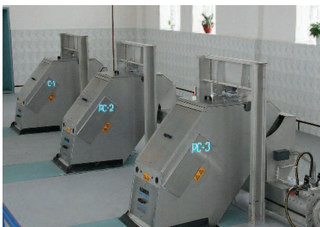
HUBER Fine Screen STEP SCREEN® SSF application in Russia: pivotable in the channel without having to remove the downstream HUBER Wash Press and HUBER Screw Conveyor.
