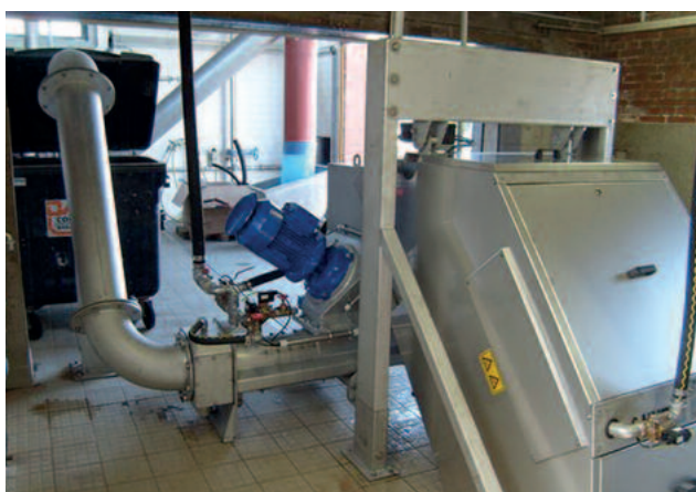
HUBER Fine Screen STEP SCREEN® SSF combined with HUBER Wash Press WAP® for intensive screenings washing. Totally enclosed, odour-free design.
