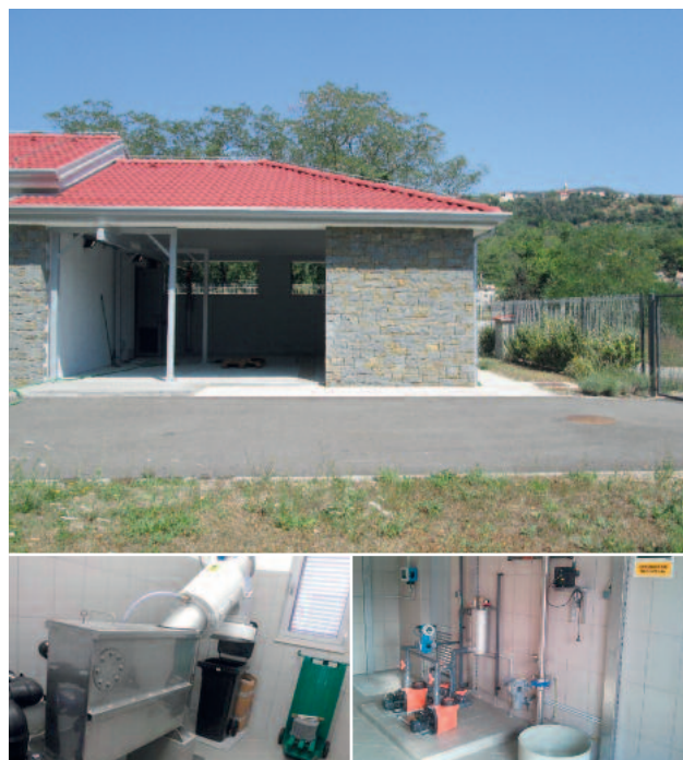
HUBER BioMem® Compact MBR system in Roc, Croatia
