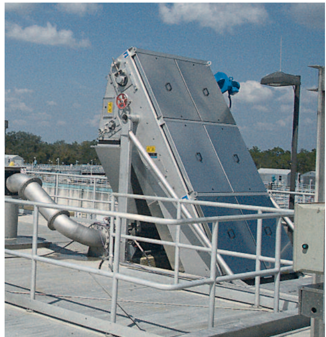
Fully enclosed, odour-free HUBER Belt Screen EscaMax® with easy to remove covers
