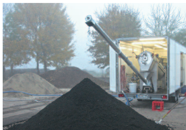
Contract dewatering with a trailer-mounted HUBER Screw Press Q-PRESS®
