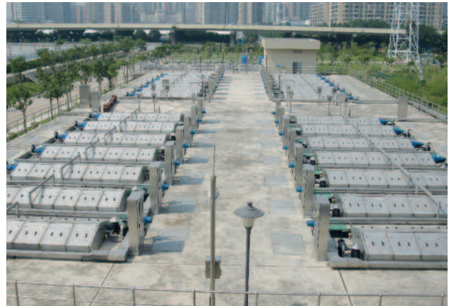
28 HUBER Disc Filter RoDisc® units with 24 discs each treating about 8.5 m 3 wastewater per second
