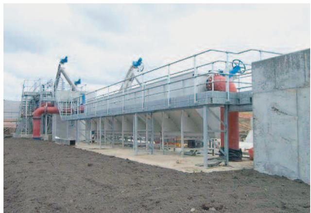
*Above-ground installation of a ROTAMAT® Longitudinal Grit Trap Ro 6 with preceding screening*
