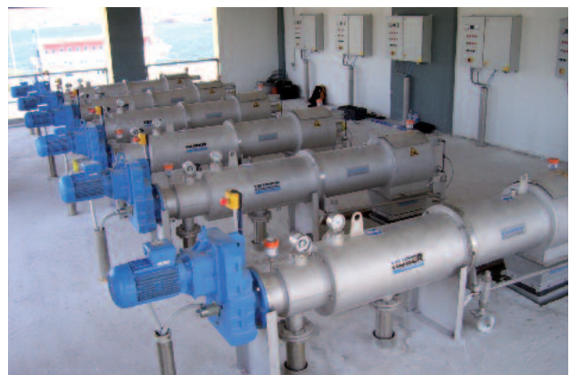
STRAINPRESS® – Continuous pressurised foreign material separation
